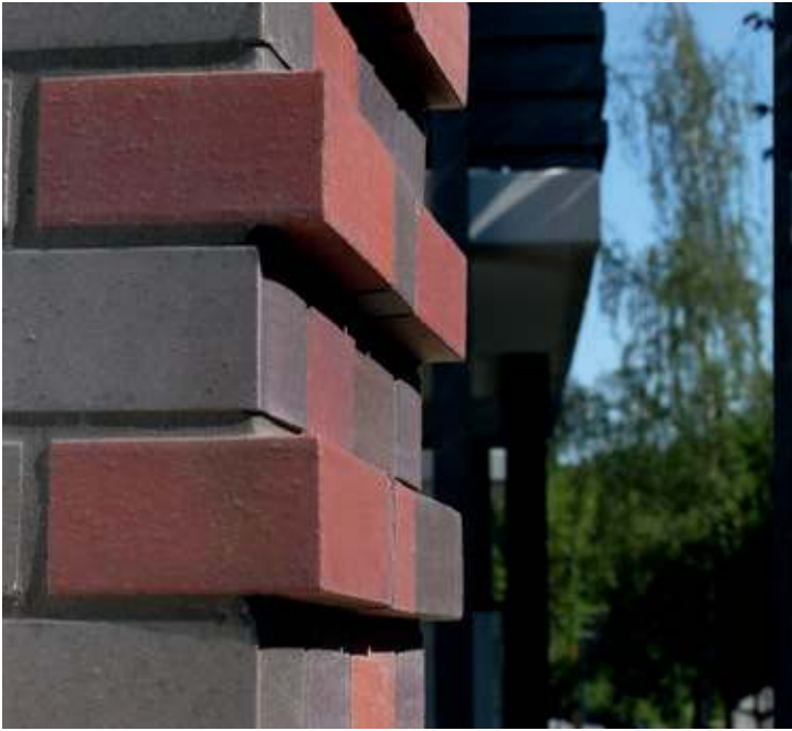
Building corner with ledge, Buchsbaumweg, Hamburg
